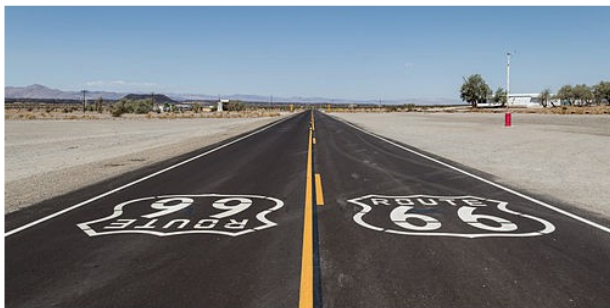
Historic Route 66 near Amboy (California, USA)
